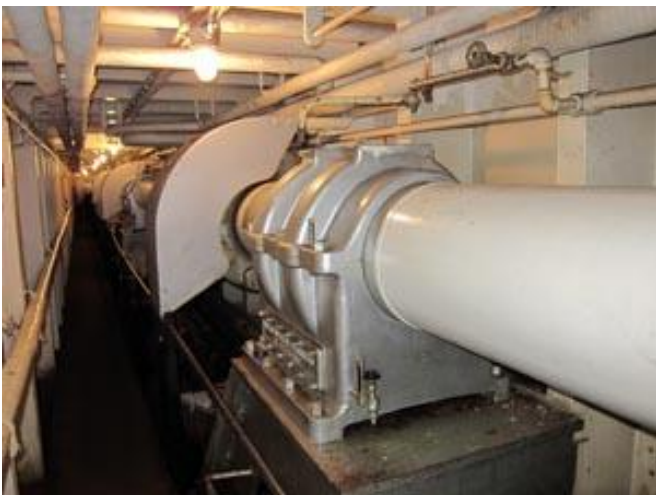
200ft Propeller Shaft Tunnel
