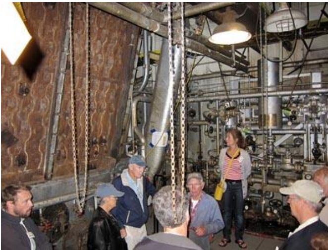
One of 2 boilers
